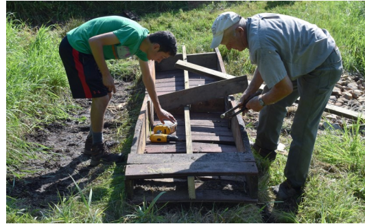
John and Jack repair the TAM's 20+ boardwalks
