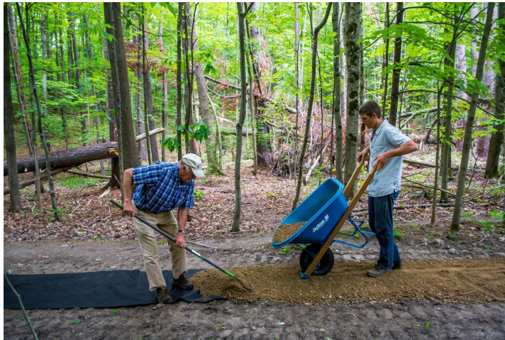
John and Caleb finish major TAM upgrades in Otter Creek Gorge
