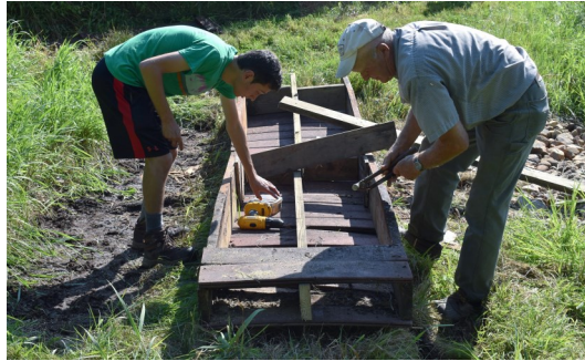
John and Jack repair the TAM's 20+ boardwalks
